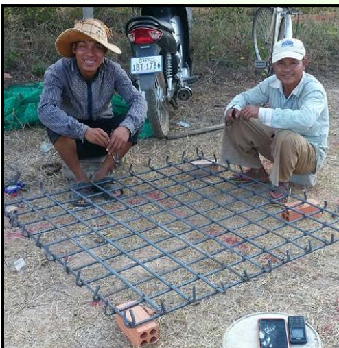
Workers preparing rebar for foundation pillars
